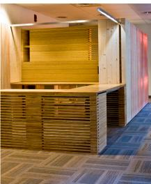
Figure 5/6: Reception wall and desk showing plywood, laminated particle board and 1"x2" strips aggregated to form surface, structure and skin
